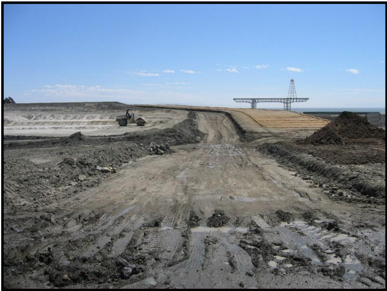
Earthmoving at Hunters Point. Source: Francisco DaCosta
