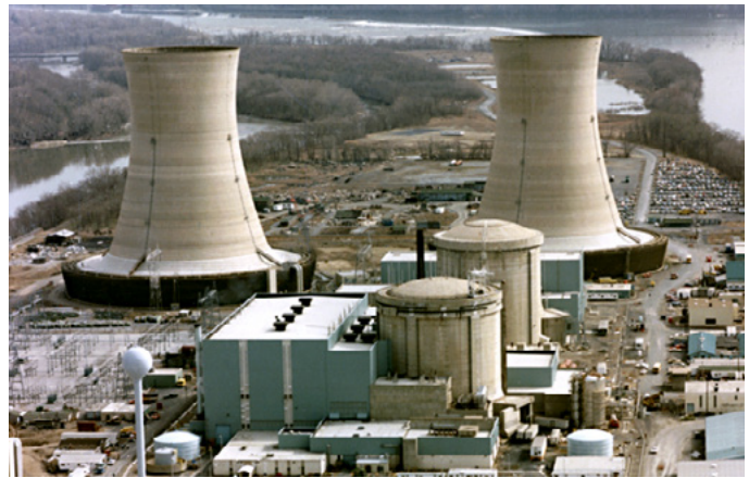
Aerial photo of Three Mile Island
