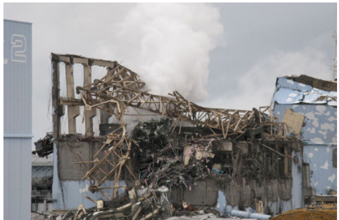
Fukushima Nuclear Power Plant Unit 3 after explosion, 2011. By Agency for Natural Resources and Energy of Japan CC BY 4.0
