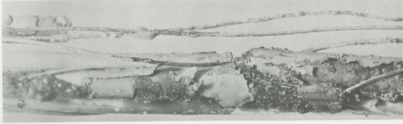
Figure IV-A-7. Midsection of Damaged Element in Channel 55
